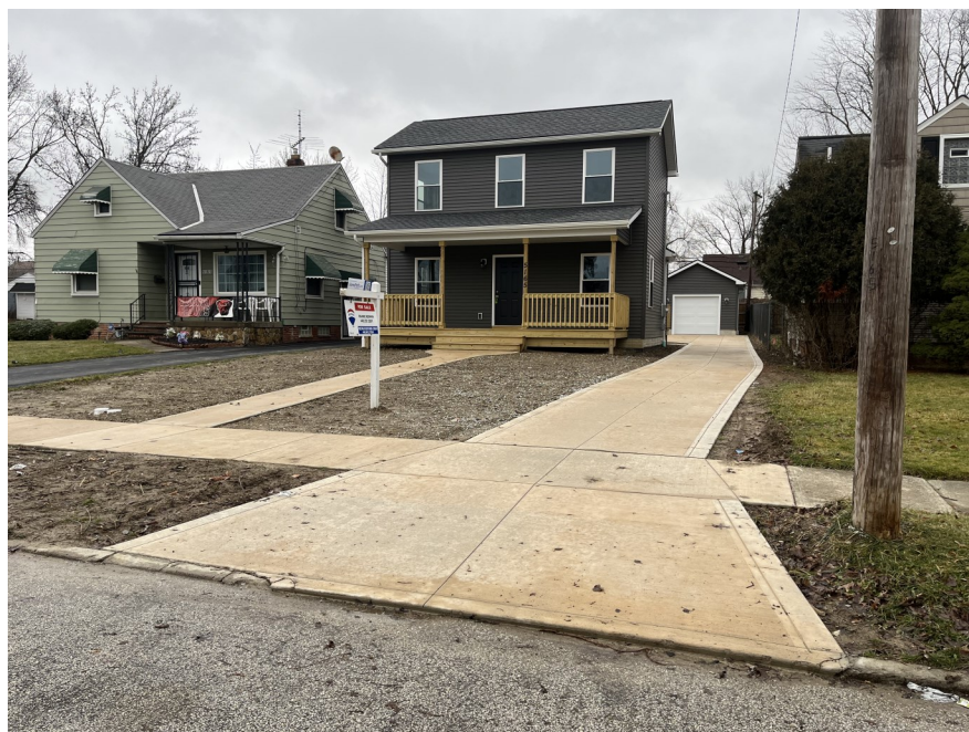
New Construction at 5165 Clement Street
