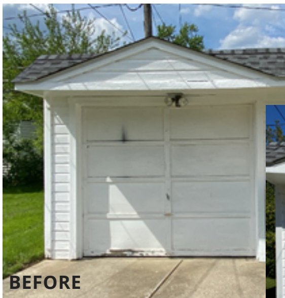
Figure 12: Repainting a Garage
