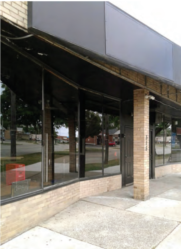
ABOVE Retail buildings along commercial are well-maintained.
