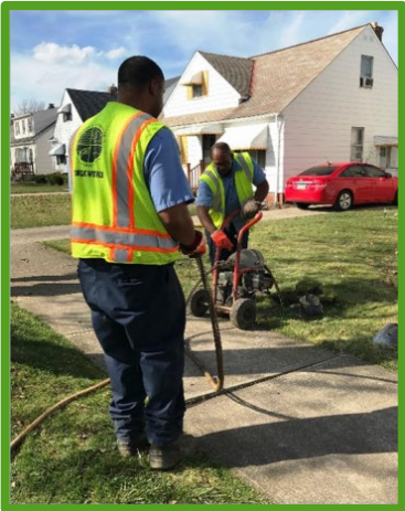
High Pressure Jet Cleaning Sanitary - 53,693 Feet Storm - 30,893 Feet
