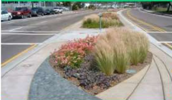
Landscaped medians can reduce pavement, slow traffic and serve as a gateway element
