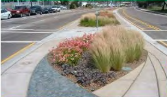
Landscaped medians can reduce pavement, slow traffic and serve as a gateway element
