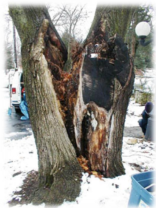
Murphy Tree- Hazard Tree ID
